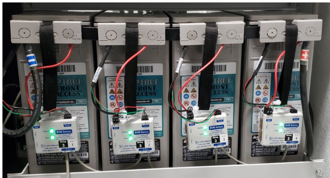
Battery sensors allow the NetGuardian to monitor your long-term battery health: voltage, temperature, and internal resistance.
