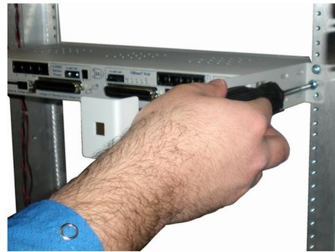
1. To begin installing the hinged pluggable back panel, the NetMediator TNT G5 should be rack mounted. **Suggestion:** Mount the unit in the flush, rack-mount position. This means the front of the NetMediator is flush with the front of the rack post.
