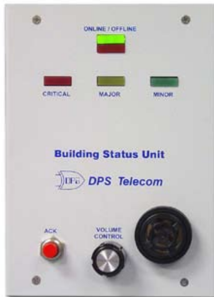
Fig. 13.1 - The Building Status Unit (BSU) shows overall facility alarm status.
